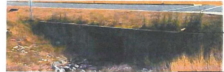
PROPOSED CONCRETE HEADWALL (MAX HEIGHT 16'). HEADWALL SHOWN IS DOTD STANDARD. DECORATIVE FEATURES MAY BE ADDED PER DEVELOPER'S DISCRETION SCALE: N.T.S.
