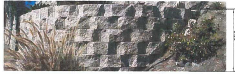
PROPOSED SPLIT FACED CONCRETE MODULAR RETAINING WALL WITH VARYING HEIGHT (MAX 5') SCALE: N.T.S.
