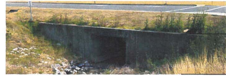
PROPOSED CONCRETE HEADWALL (MAX HEIGHT 15'). HEADWALL SHOWN IS DOTD STANDARD. DECORATIVE FEATURES MAY BE ADDED PER DEVELOPER'S DISCRETION SCALE: N.T.S.
